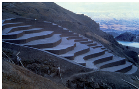
Stabilisation of landslide - Cairmuir (New Zealand)
