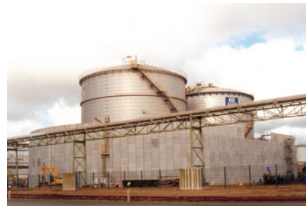
Containment dikes for ammonia tanks - Montoir (France)
